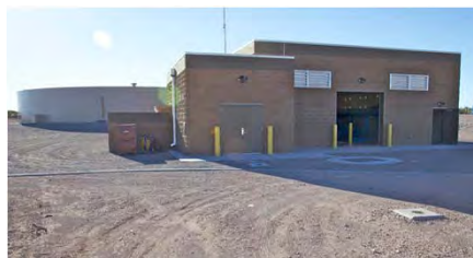
1.3M gal Water Storage & Booster Station
